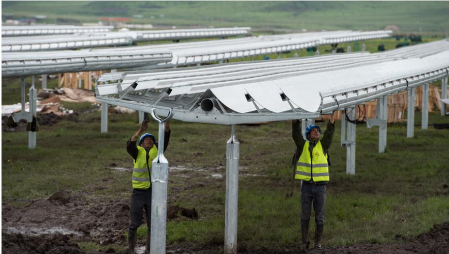
Workers install panels at a solar station in Hongyuan, China, in June 2015. Photo by: Jie Zhao/Corbis via Getty Images
